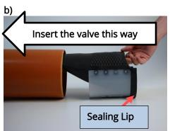
b) Insert the valve until the sealing lip is completely fitting inside the pipe. When inserted correctly, the valve should sit within the pipe as shown in picture (c).
